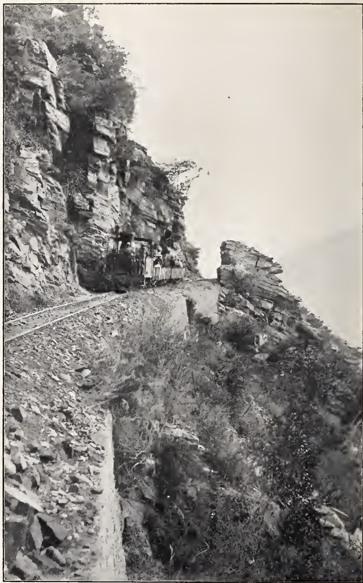
A PIECE OF THE CONGO STATE RAILWAY
